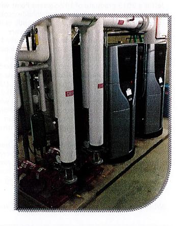
to new, more reliable high-efficiency, condensing boilers. In addition to the boilers being identified for replacement, much of the original 1974 pump configuration was obsolete due to new technologies and was also targeted for clean-up.
