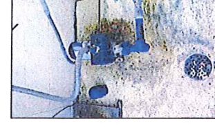
6 CHLORINE BOOSTER PUMP R-M1 TO BE REPLACED
